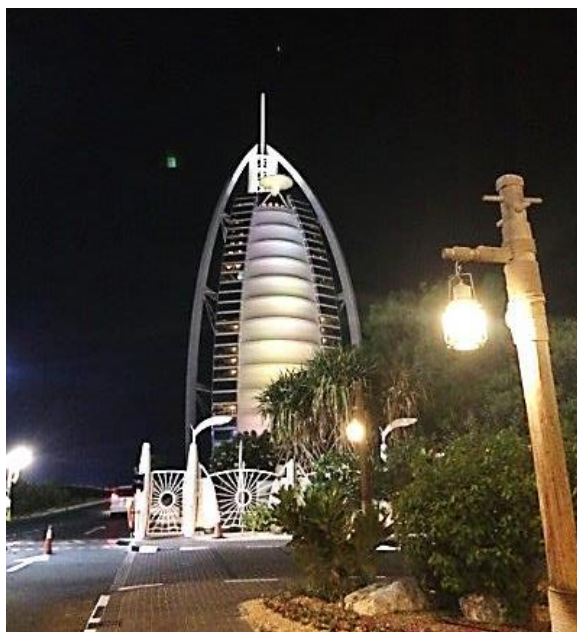
Figure 12: Guarded and gated bridge leading to Burj Al Arab (Author, October 2015)
